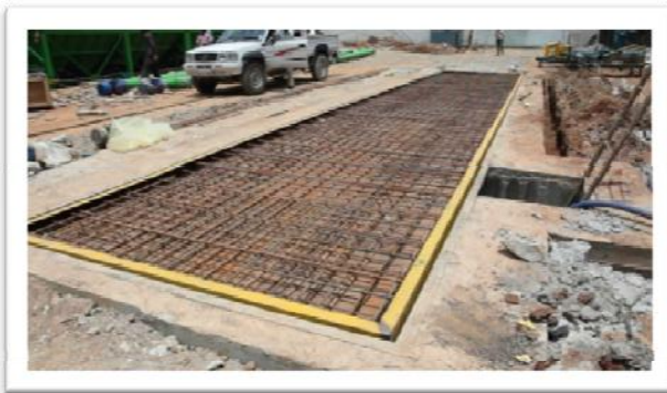
4. Laying of Re-enforcement
