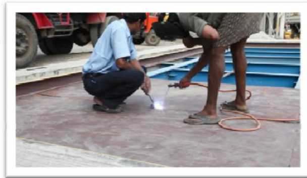
3. Welding of Base Sheets
