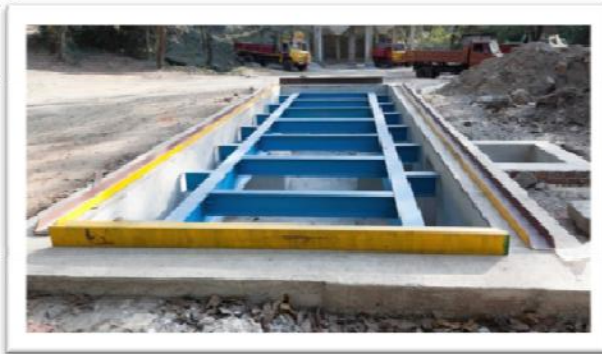
2. Assembly of Beams
